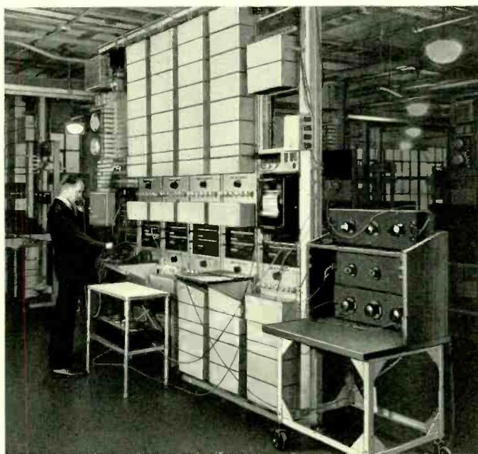
*Fig. 2—G. P. Wennemer at a cable carrier-telephone terminal in the carrier laboratory on the 10th floor*
