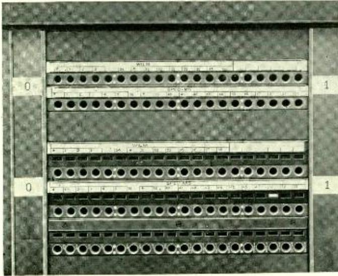
Fig. 3—The new busy strip, employing the E-1 lamp, occupies only half as much vertical space as the former magnetic type of signal
