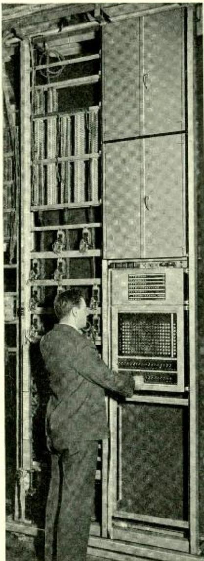
*A standard test circuit for subscriber's senders in the systems laboratory*
