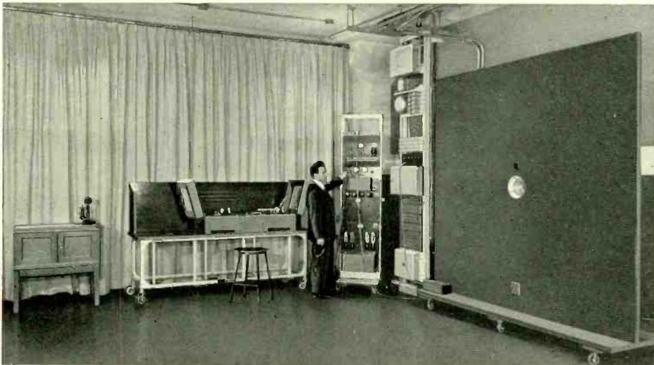
*Fig. 5—Walls of the program observing room have been treated with rock wool to obtain a desirable reverberation time which may be varied by adjusting monk's cloth curtains at one end. In the background is a phonograph-reproducing set and on the right is a high quality loud speaker with baffle board*
