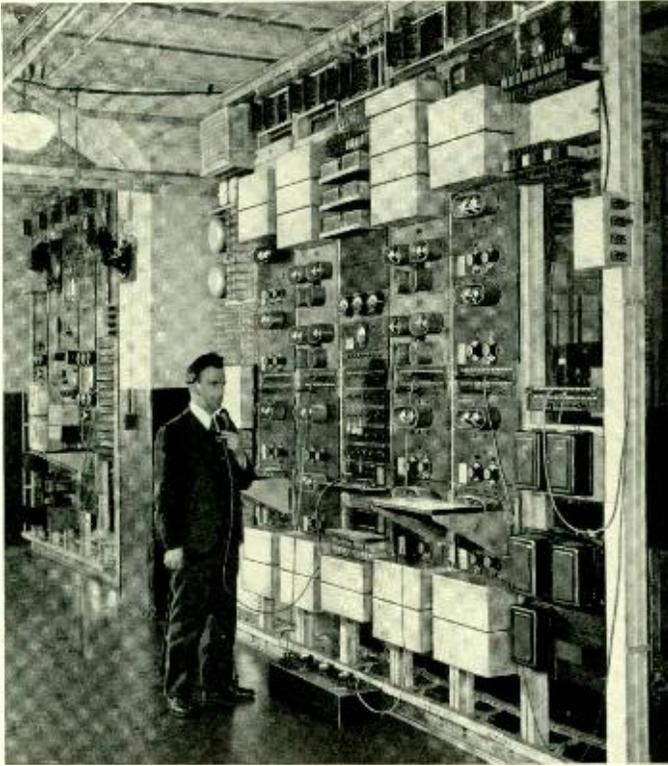
*Fig. 3—F. A. Muccio at one terminal of a Type-C carrier-telephone system*
