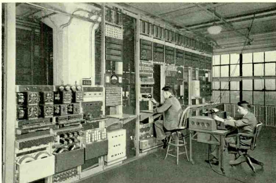
*Fig. 1—R. G. Loeffel, left, and C. A. Dahlbom with grounded telegraph equipment and open wire repeaters in the telegraph laboratory on the 11th floor. The fourth bay from the left is one of the permanent power panels*
