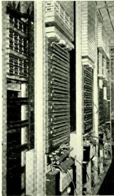
*Fig. 5—A partially completed installation of relay-rack equipment to be associated with busy lamp signals*
