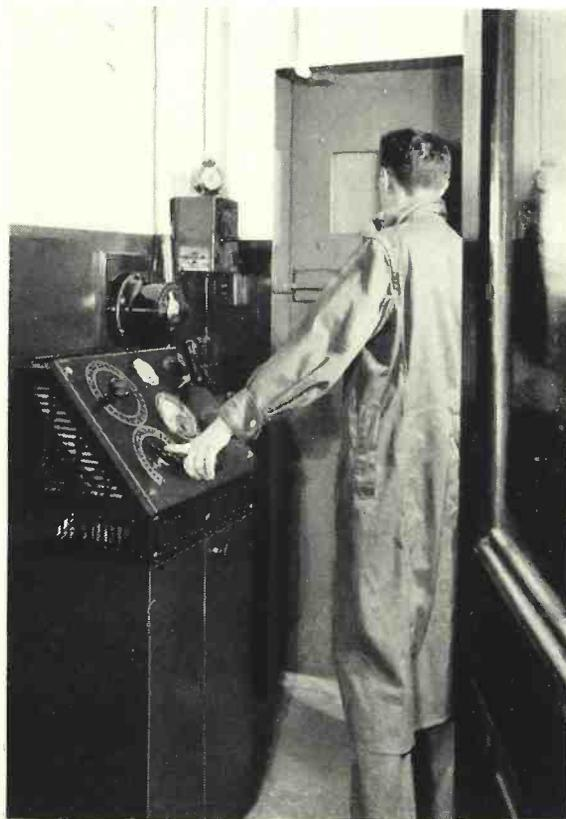
*Fig. 5—The X-ray apparatus is controlled from an outer chamber. A lead-glass window permits the operator to view the interior of the X-ray room as he stands at the controls*
