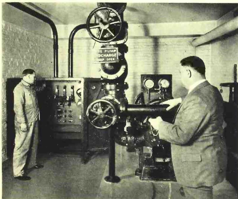
*Making a periodic test of the 1,000 gallon electrically driven pump. Fire Inspector William Wissel observes the pressure gauges after the switch is thrown by W. C. Somers, in charge of the power plant.*
