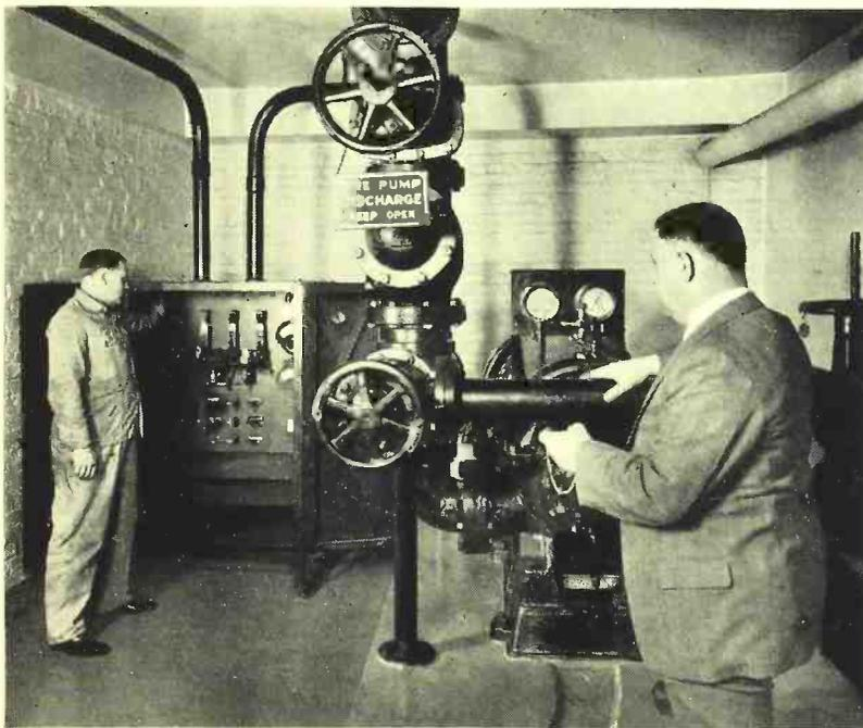
*Making a periodic test of the 1,000 gallon electrically driven pump. Fire Inspector William Wissel observes the pressure gauges after the switch is thrown by W. C. Somers, in charge of the power plant.*
