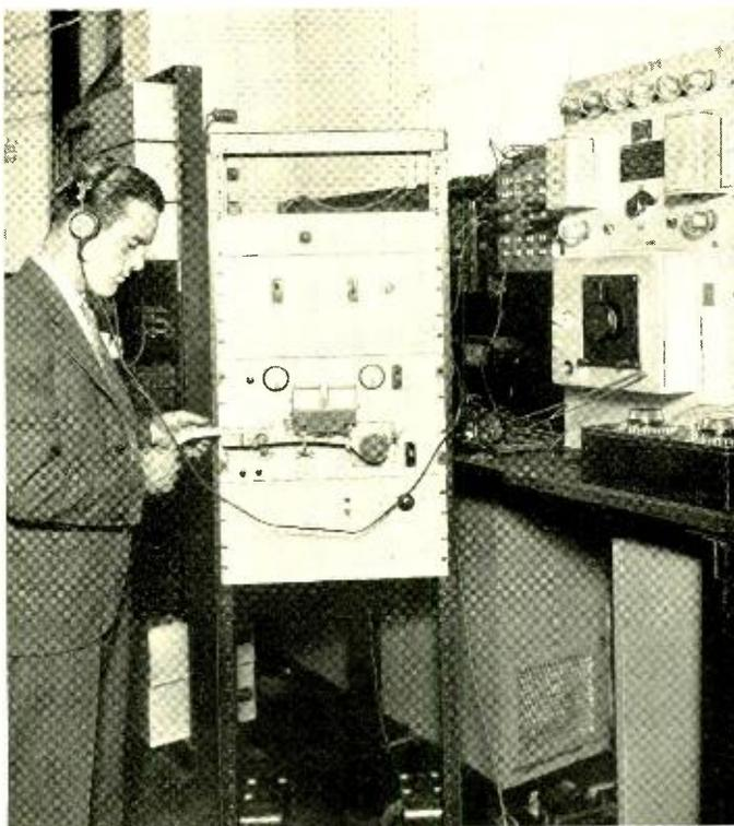
Fig. 2—The author reading the automatic level recorder used in the measurement of the transmittivity of walls
