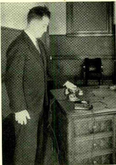
*Fig. 2—A small receiving set has been developed to measure the transmission loss of subscribers' lines. By calling a designated number, P. F. Jones has automatically connected the 1000-cycle generator to the other end of the line and is about to read the meter*
