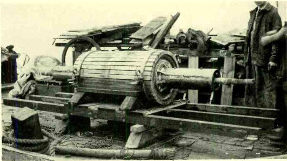
*Fig. 5—The new submarine loading coil case ready for installation*
