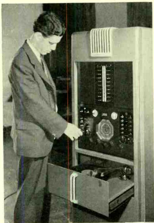
*Fig. 1—The new program sound system comprises a radio receiver, a phonograph and three microphone input circuits*
