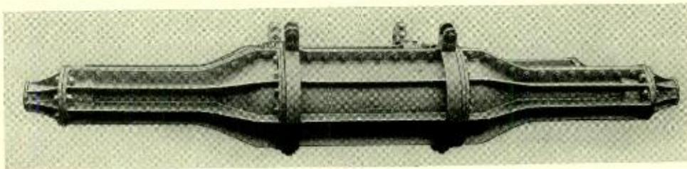
Fig. 2—The early loading coil case was sixteen feet long and weighed nearly five tons
