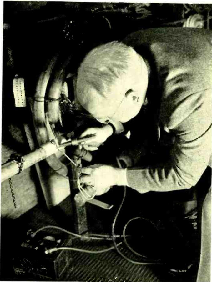
*A method of repairing ring cuts on cable sheath, using a carbon-electrode soldering outfit, is demonstrated in the laboratory by V. B. Pike*
