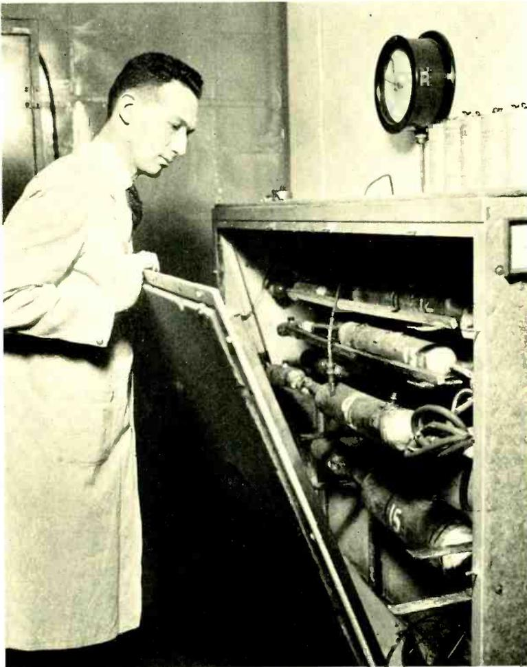
*Several specimens of pressure-testing plugs are being subjected by H. Baillard to life tests at elevated atmospheric temperatures*
