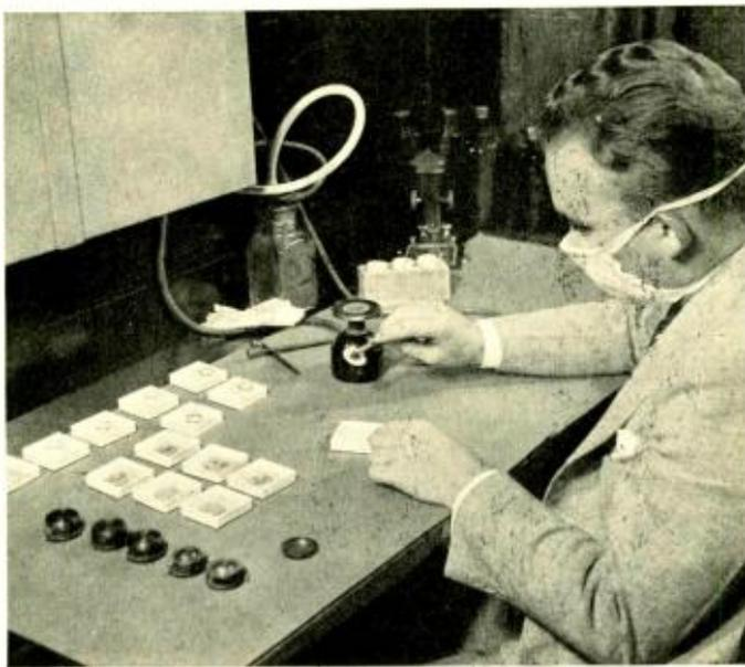
*Fig. 1—A special suction tool permits the diaphragm to be handled during assembly without touch by the hand*
