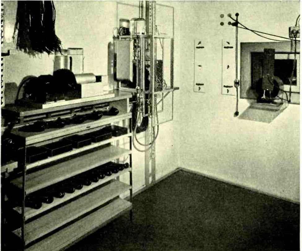
*Fig. 1—The temperature and humidity of this test room, used to determine the effect of moisture on telephone apparatus, are accurately controlled by the vapor-pressure thermostat and humidostat shown mounted on the left wall beyond the apparatus rack*
