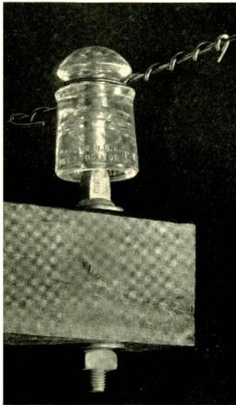
*Fig. 2—Insulator, CS type, with steel pin and lead thimble*
