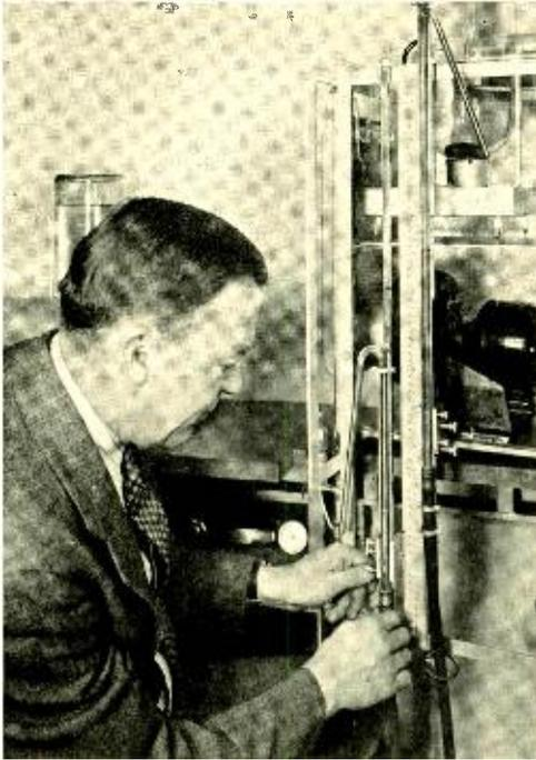
Fig. 2—W. A. Bunzel adjusting the vapor-pressure thermostat and humidostat
