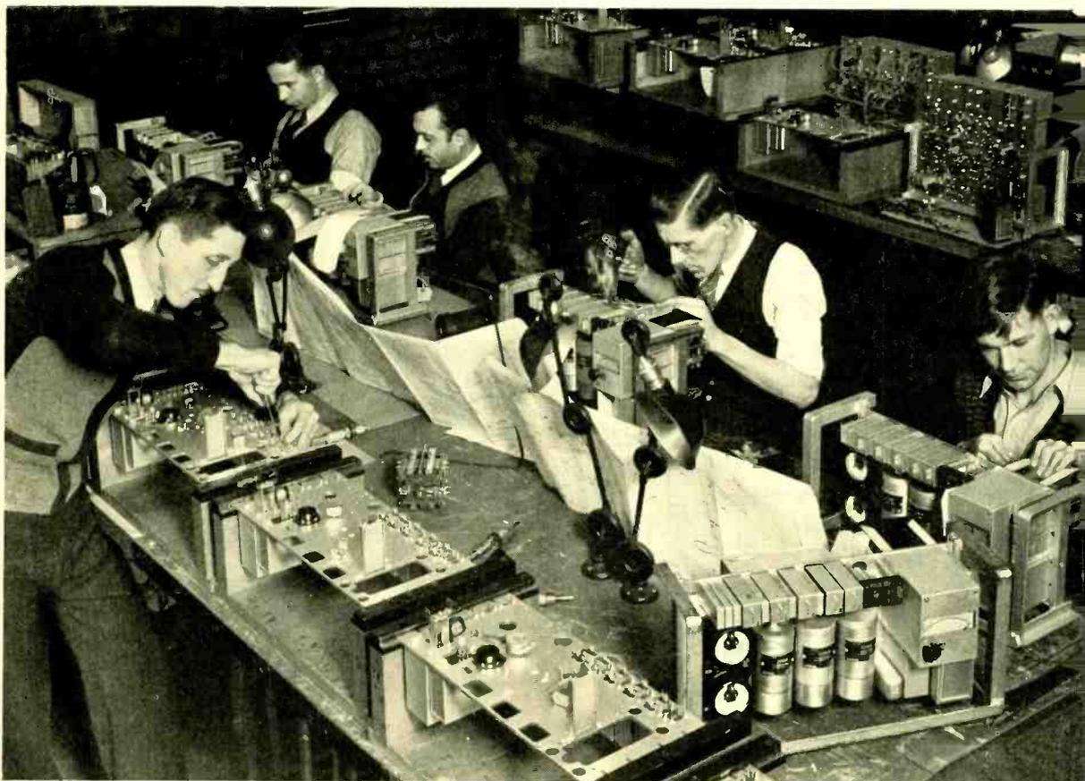
2B Regulators are assembled and wired at the Kearny works of the Western Electric Company. The characteristic curves below show (a) varia-
