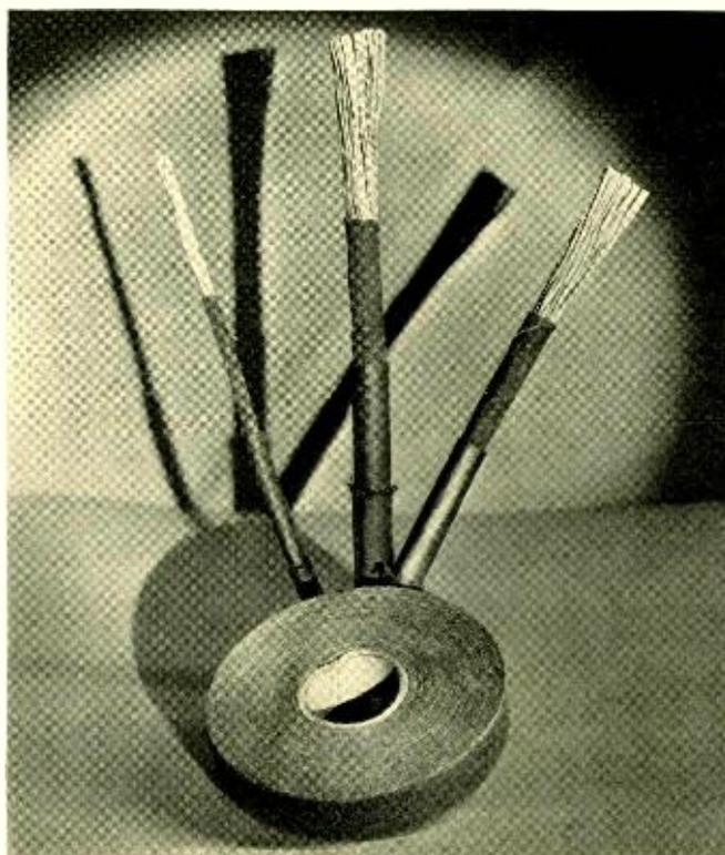
*An improved cable for inside wiring which has better moisture-resisting characteristics than similar cable now in use is shown here. The improvement results from the addition of a thermoplastic jacket between the core of the cable and the braid. This jacket makes unnecessary a cord under the braid to aid in stripping; and it permits the cable to be made with a smooth surface and more pleasing appearance.*
