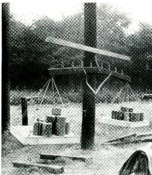
*Breaking tests on crossarms at the Chester field laboratory. Test arms were loaded with weights*
