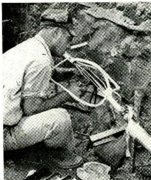
*Splicing a coaxial cable now being laid between Atlanta and Jacksonville*
