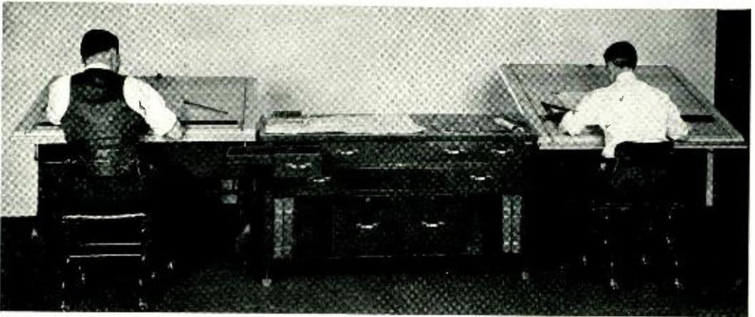
*Between each two drafting boards there is a storage cabinet for drafting tools, drawings and reference books. The boards, themselves, are adjustable from horizontal to vertical and also for height by easily operated levers. They can be set at any desired elevation from desk level to a height convenient for the draftsmen to work while standing*
