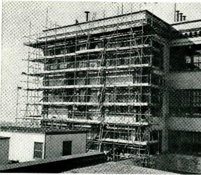
*This photograph shows major repairs being made on Section A—required by the corrosion of steel which was caused by leakage of moisture through the brickwork over a period of forty-five years. Pointing up the masonry and other methods used in the past had retarded but not prevented this corrosion*
