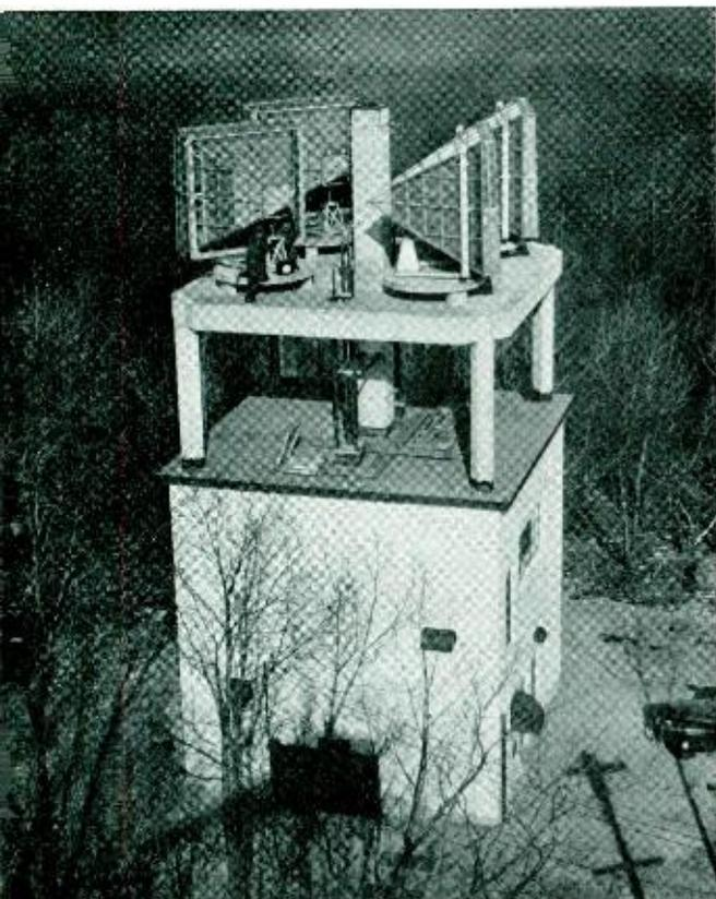
Fig. 2—One of the repeater stations of the New York-Boston system showing antennas on the roof
