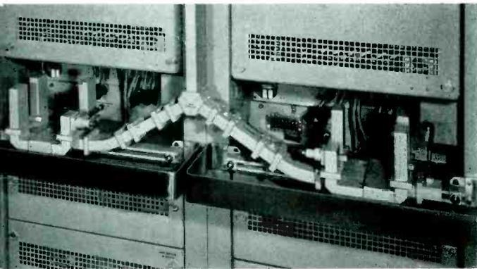
Fig. 5—Close-up view of transmitting waveguides
