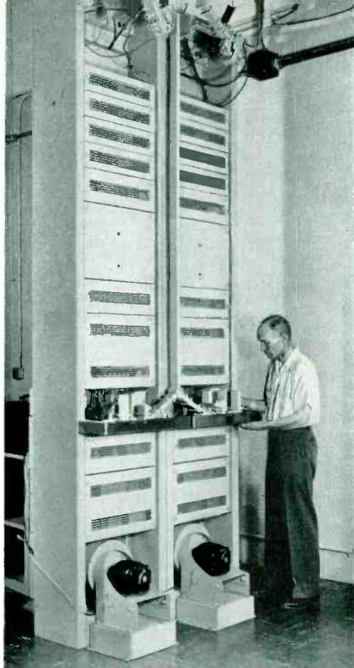
Fig. 4—Front (left) and rear views of two relay bays at a repeater station
