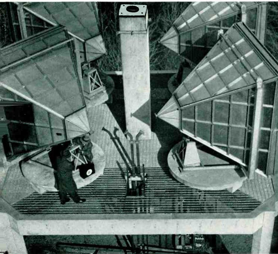
Fig. 7 - Antenna platform of Jackie Jones station showing antenna plates and the floor of subway grating
