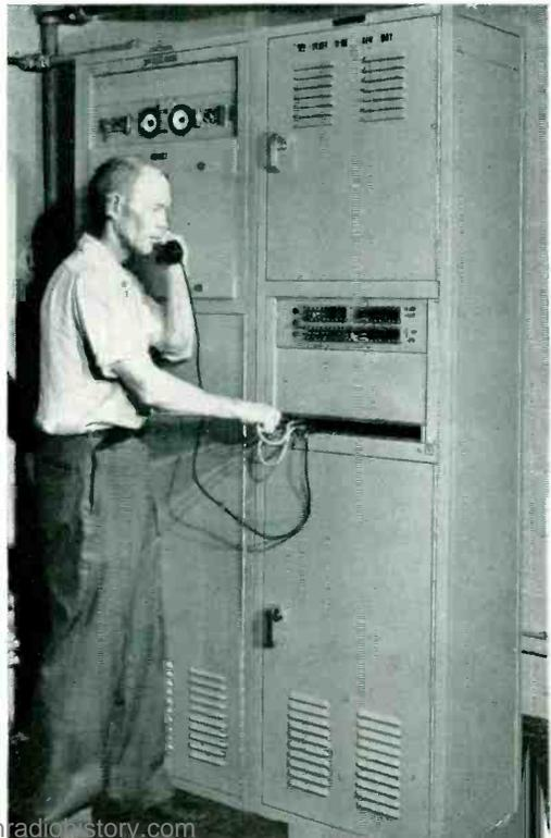
*Fig. 10—24-volt power control cabinet and order-wire and alarm cabinet on the second floor of the repeater station*
