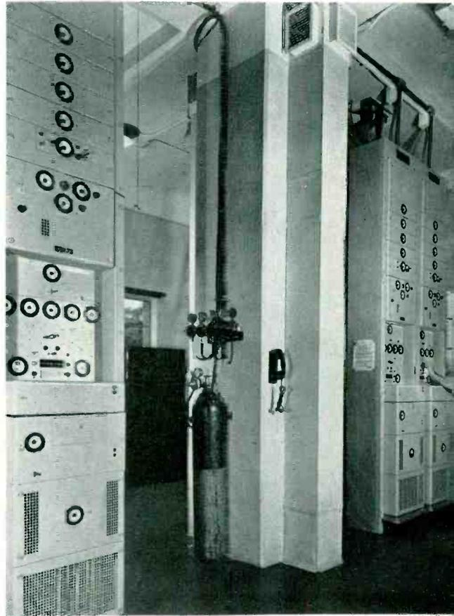
*Fig. 9—Second floor of a repeater station showing the repeater bays at each side of the central column*
