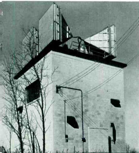
Fig. 3—Right side, at left, and rear of Bald Hill station. Low wall opposite rear of building is to prevent back-drafts to the engine exhaust
