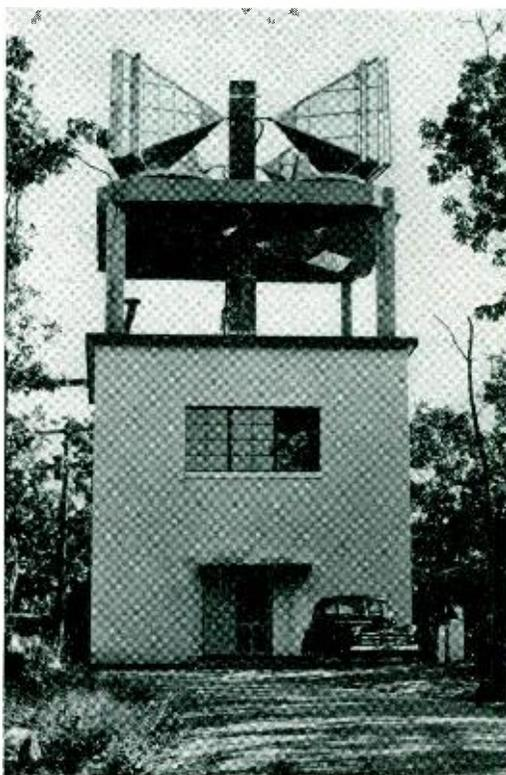
*Fig. 11—Front view of Birch Hill radio relay station. This and the Jackie Jones station have antenna platforms 14 feet above the roof*
