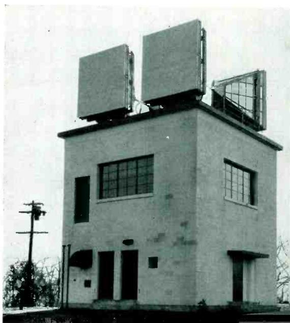
*Fig. 2—Front, at the right, and left side of Bald Hill station. The two doors on the left side lead to the engine and furnace rooms*
