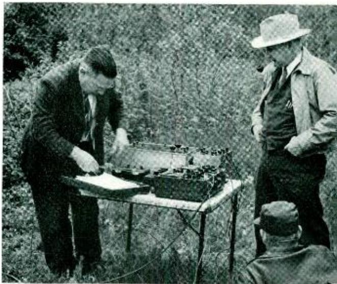
*Trial of new equipment for corrosion testing on the Catskill-Albany underground cables. Robert Pope at the instruments, T. J. Maitland (Long Lines) and J. H. Harding in foreground*
