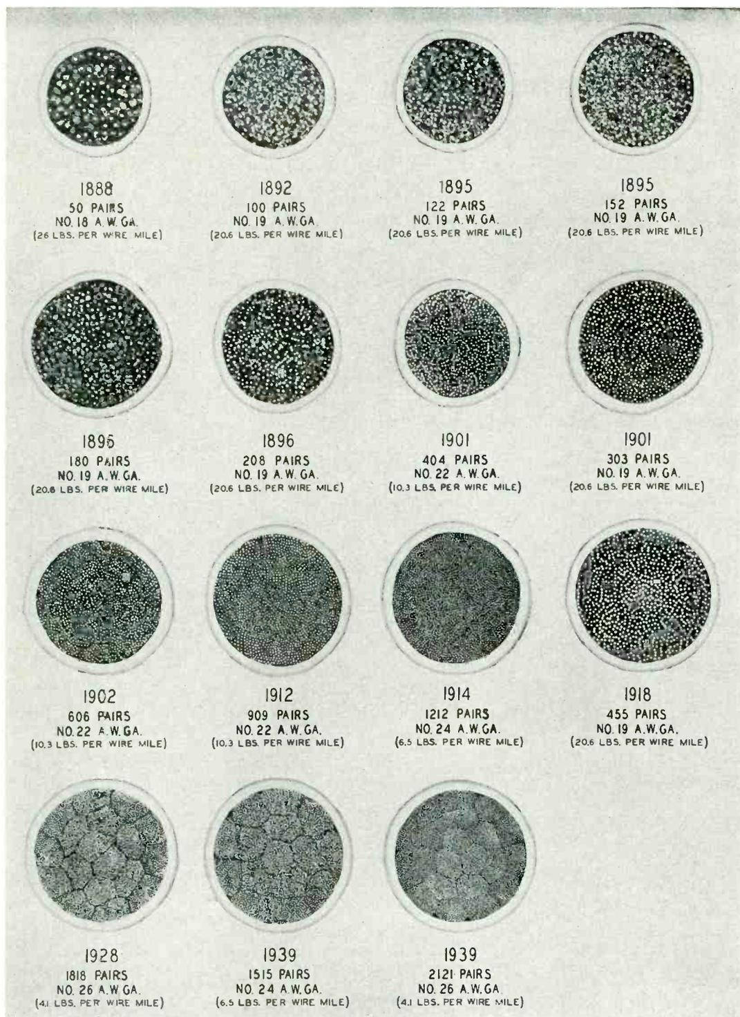
Fig. 3—A pictorial survey of full-sized Bell System exchange cables from the first paper-insulated lead-sheathed cable of Barrett's to the 2121 pair cable of 1939. Cables in the two bottom rows are 2½ inches outside diameter
