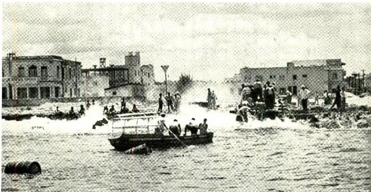
*Fig. 2—Oil drums supporting the cable were pulled onto the coral Cuban beach by a winch. This location is about five miles from the center of Havana.*
