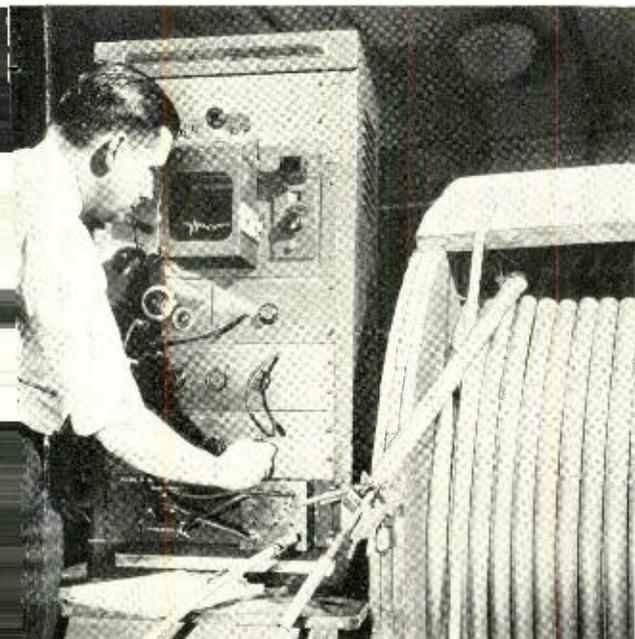
Fig. 1—Operating a field set to obtain pulse echo measurements.
