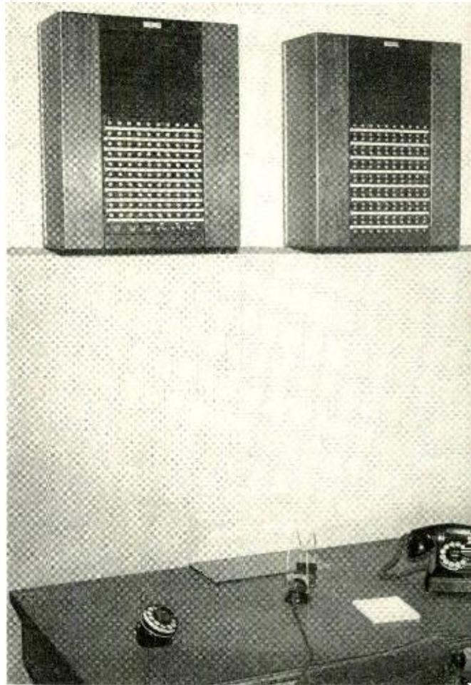
Fig. 5—A supervisor's position showing two lamp cabinets.
