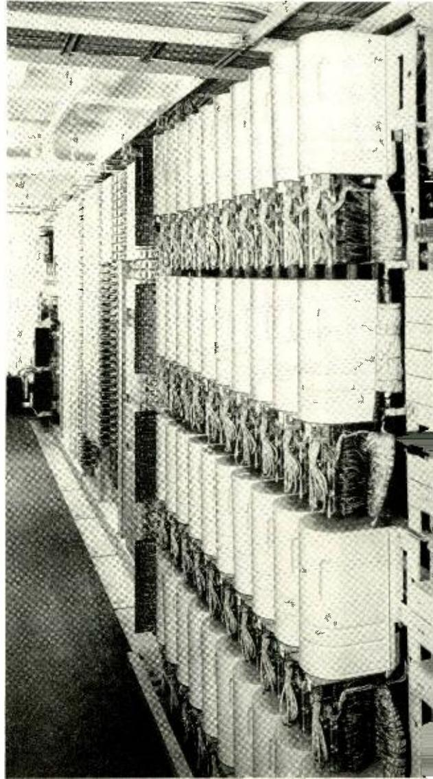
Fig. 6—Switching equipment for the 6A order turret.
