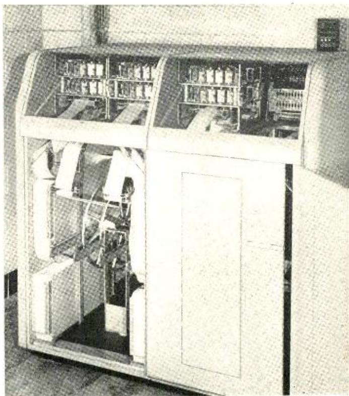
*Fig. 2—Two tape perforators with their supplies of used and unused tape are mounted in a single cabinet.*
