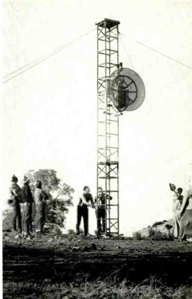
Part of the job of creating a microwave relay route is the survey which tells whether there is a satisfactory line-of-sight transmission path between two proposed station sites. It is made by setting up portable towers developed in the Laboratories (RECORD, January, 1948, page 6) and running a movable antenna and reflector up and down. These pictures were taken by G. M. Eaton of the Pacific Company.
