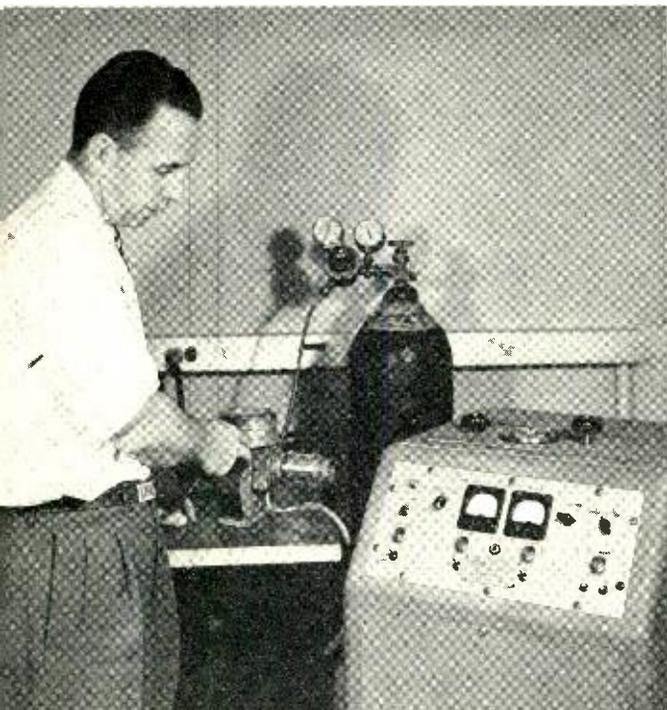
Fig. 4—E. D. Morris testing a 1555 magnetron with the helium leak-detector.
