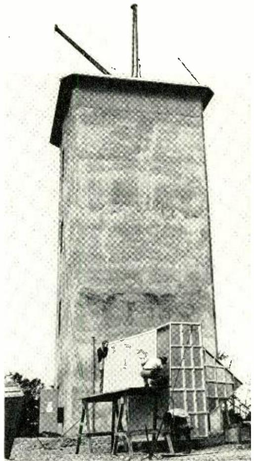
*Fig. 7—A lens being assembled on the ground preparatory to hoisting to tip of tower.*
