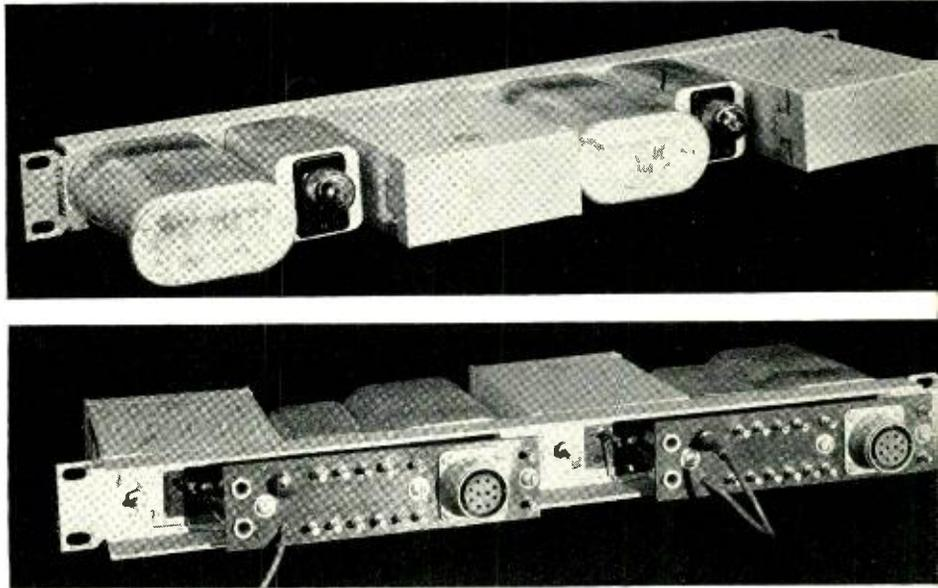
are no line jacks for patching the repeater, and there are no variable gain controls, the gain being determined by the network strapping. Neither filter units nor equalizer units, as are required in other repeaters, are used with the E1 because these features are built into the amplifier and network circuits. No additional equipment is required. Thus, the only external wires required for the repeater are two pairs of line conductors and four wires for connection to the power supply.
