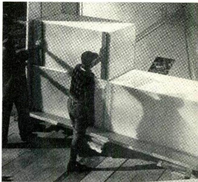
Fig. 6—Placing the lens section in the housing.
