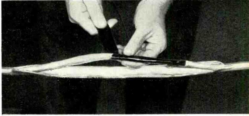
*A strip of lead serving-tape is inserted in the opening to give a base for solder and also to re-enforce the cable at the repair line.*
