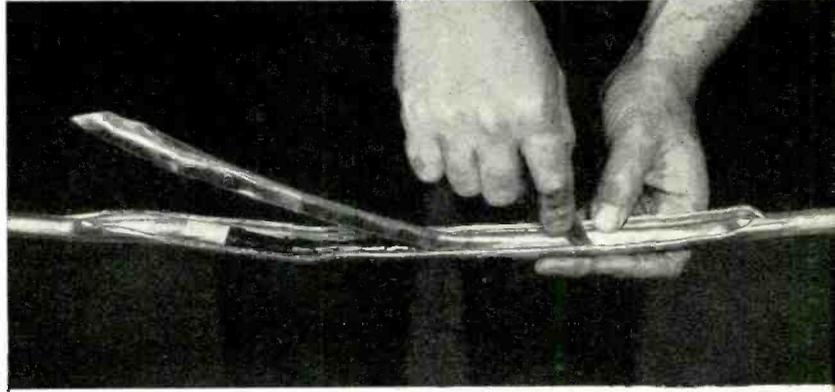
*Closure of the sheath around the core restores as closely as possible the original contour of the cable.*
