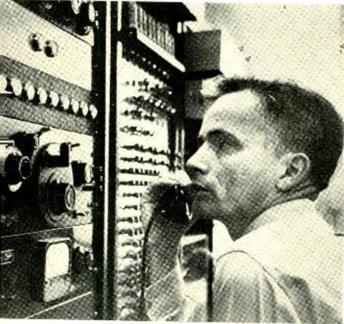
*An electronic telephone device which can understand and intelligently react to spoken numbers is put through its paces by K. H. Davis. "Audrey," as the device is known, has a special circuit which automatically determines which of ten numbers has been spoken into an ordinary telephone, and flashes an appropriate light.*
