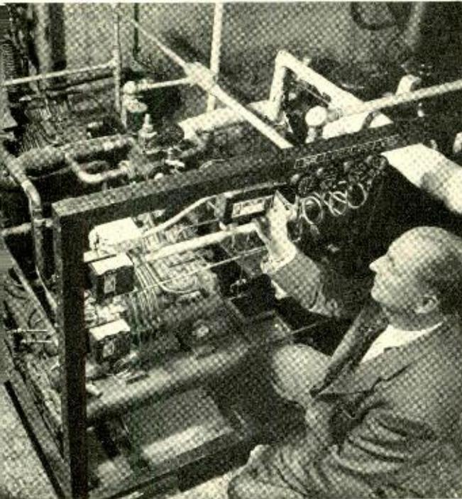
Fig. 2 — The refrigerating plant consists of a single 10 hp stage, at the right, and a secondary stage comprising two 3-hp units at the left. The author is checking the operation of the plant.
