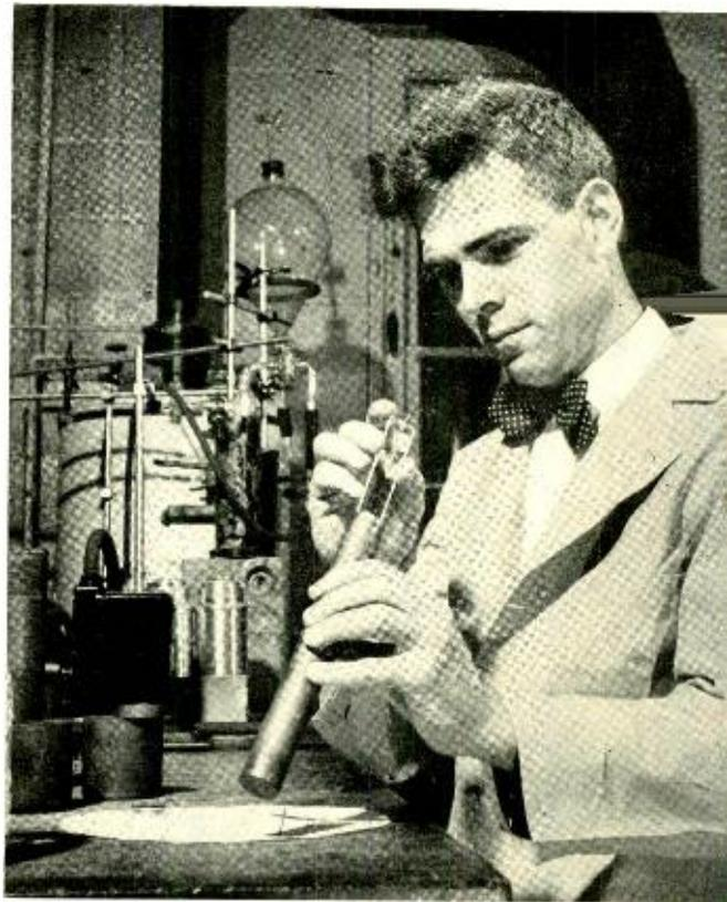
*Fig. 5—Loading seed-crystal plates into the inner liner of an autoclave.*
