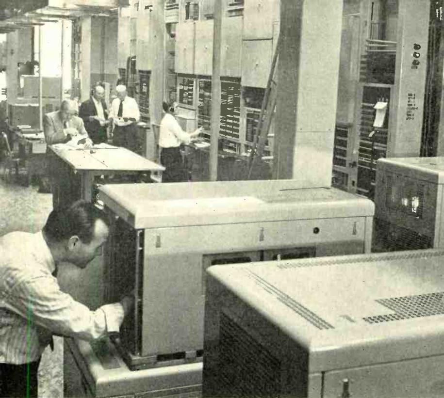
*Fig. 3—Part of a 4A sectional center showing a group of card translators in the foreground and another in the background (left) with the maintenance center between them.*
