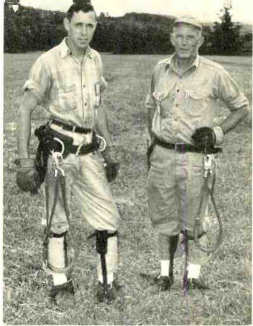
*On the ground, the cushion body belt worn by the man on the left rides easily and comfortably. The name comes from the five-inch wide "cushion" of leather next to the workman's body.*
