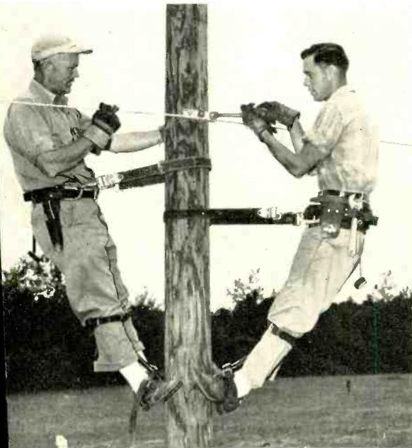
*Aloft, the cushion body belt provides a soft cushion about the hips, preventing chafing or abrasions possible under extreme weather conditions or during long working periods. The man at the left wears the body belt normally provided.*
