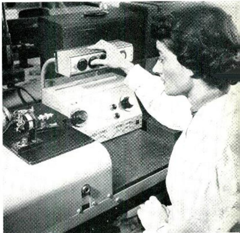
*Fig. 3 — Mrs. Claire Briede at Bell Telephone Laboratories using a machine developed by the Western Electric Company to wind a 436A grid.*
