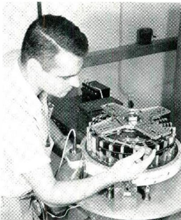
Fig. 8 — J. J. Moran at a dividing head for adjusting potentiometer brushes. Shown is a large spiral potentiometer, containing a ninety-inch card and brushes that move radially as mounting rotates.
