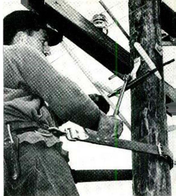
*Fig. 6—Telephone lineman placing new rural distribution wire using reinforcing strap for pole attachment.*
