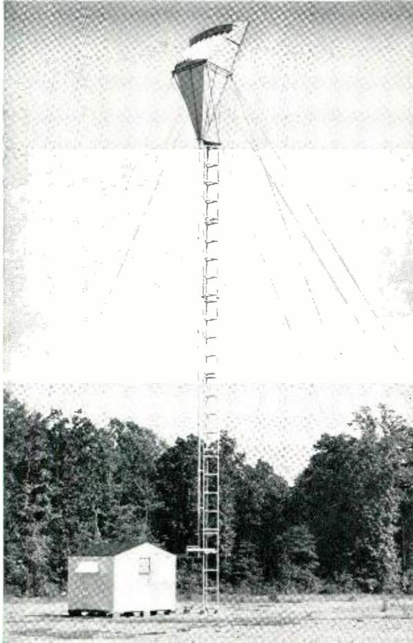
*A developmental model of the new radio relay antenna at the Holmdel Laboratories.*
