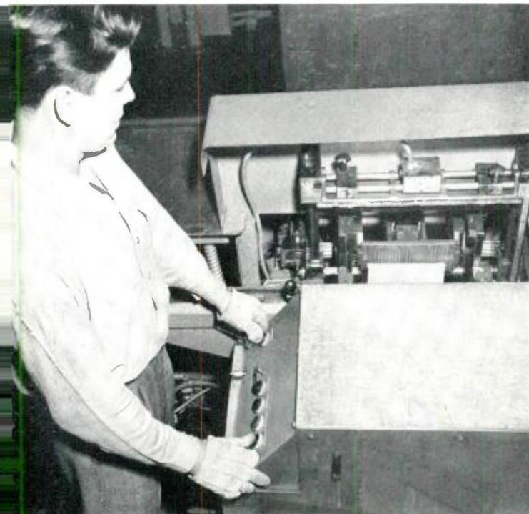
*Fig. 4 — The molds are stripped from the cast terminal strip by this machine, operated by V. H. Cullum.*
