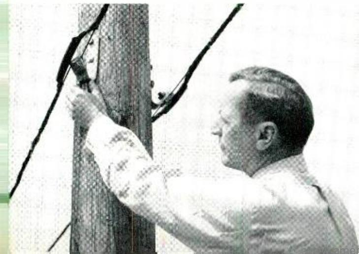
below the crossarm. In attaching the crossarm type bracket, the long leg of the "J" is placed against the side of the crossarm, with the end extending somewhat above the arm. The bracket is fastened in place with a "U" bolt which spans the arm. This method of fastening avoids having to drill the crossarm and prevents rotation of the bracket. A lag screw, driven into the side of the crossarm through a hole in the bracket, prevents lengthwise movement along the arm.
