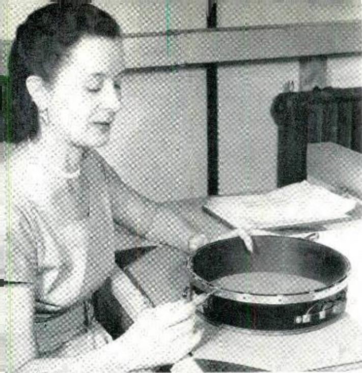
*Fig. 3—Miss Motowska here makes an adjustment on a card and drum assembly. Scallops in card permit accurate alignment of calibrated points on card with fiducial marks on drum. In many cases the circumference is shared by three or four cards.*
