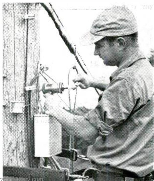
cable, heating asphalt and handling hot material, and making constrictions in the sheath. Tools and materials for the resin method are light in weight, compact, and can be carried up the pole in pouches attached to the body belt of an individual workman.
