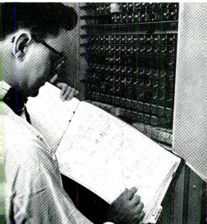
Fig. 4—J. M. Sangster, equipment maintenance man, using a functional schematic at the Long Lines No. 4 cross-bar office in New York City.
