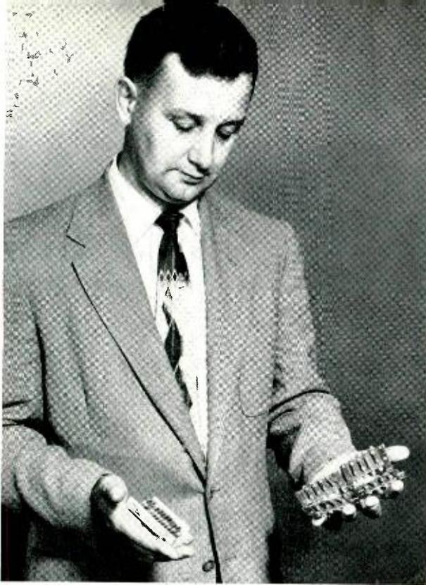
*Fig. 1—W. T. Westaway compares a Minaplas assembly for A4 channel banks with the previous terminal cards.*
