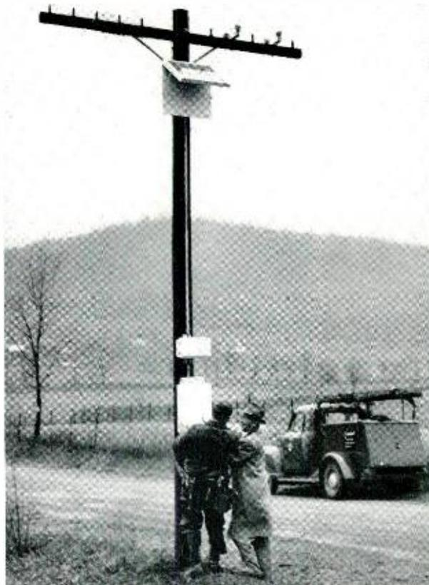
*Among the photographs in the 1954 Annual Report was this picture of a “mock-up” Bell Solar Battery as it would be used to furnish power to a rural telephone line. Shown in the picture are F. W. Bingert, left, of the New Jersey Bell Telephone Company and A. C. Kane of Bell Telephone Laboratories.*
