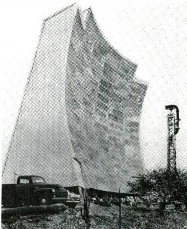
*A 60-foot parabolic reflector for receiving and sending radio waves “over-the-horizon.”*
