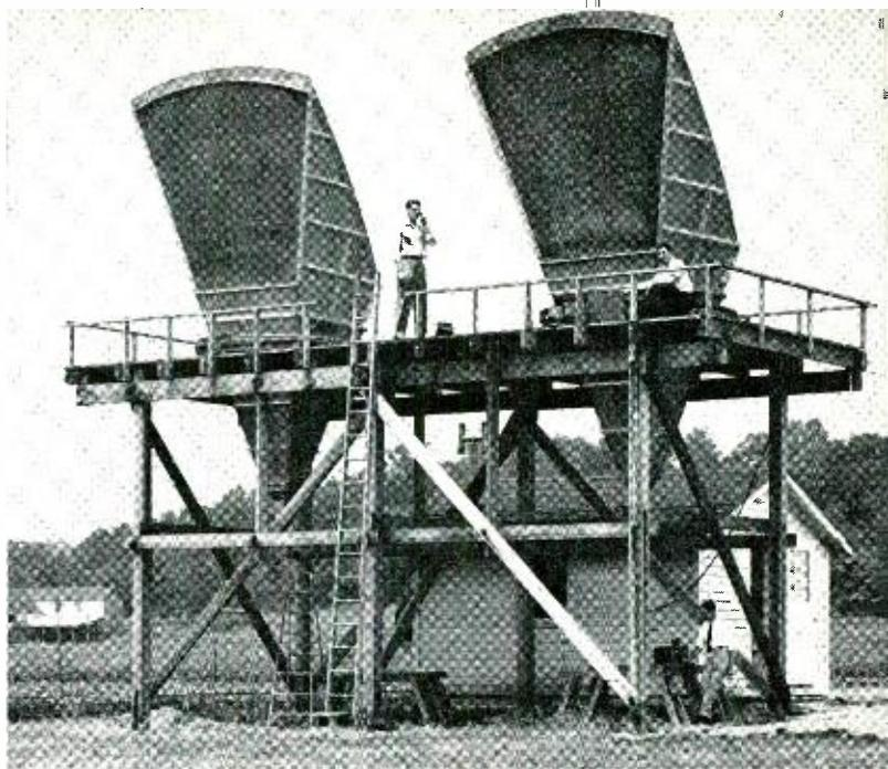
1,000,000,000,000 to 1 is the ratio of power transmitted by one of the antennas, shown above, to the level of crosstalk received by the adjacent antenna. Measurements of this magnitude can be made with equipment employing radar pulse techniques. Useful not only in measuring antenna performance characteristics, but also in accurately evaluating minor changes in design, this pulse test equipment has contributed to the development of improved antennas for "backbone" microwave routes.
