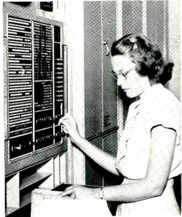
Fig. 2 — Miss Betty Boyd putting problem information into the Bell Laboratories Model V relay computer. These early computers used electromechanical computing elements, and required large rooms full of relay racks for their operation.
