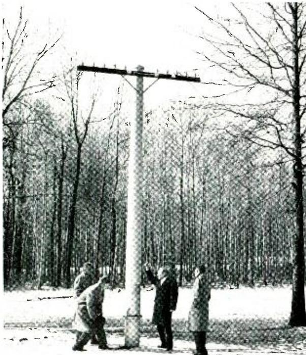
Fig. 4 — This telephone pole is hollow and contains a thermoelectric generator of one-watt capacity powering a transistor amplifier. The lower portion of the pole is a storage tank for "bottled gas" used to operate the generator.
