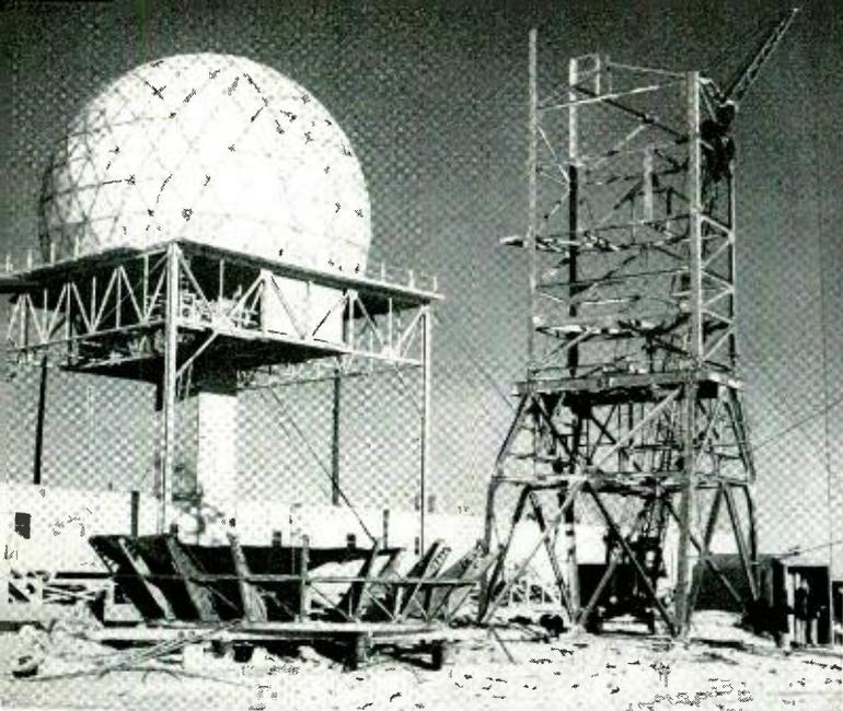
*Fig. 3 — Reflector being assembled on the ground at a snow-covered DEW Line site in the Arctic.*
