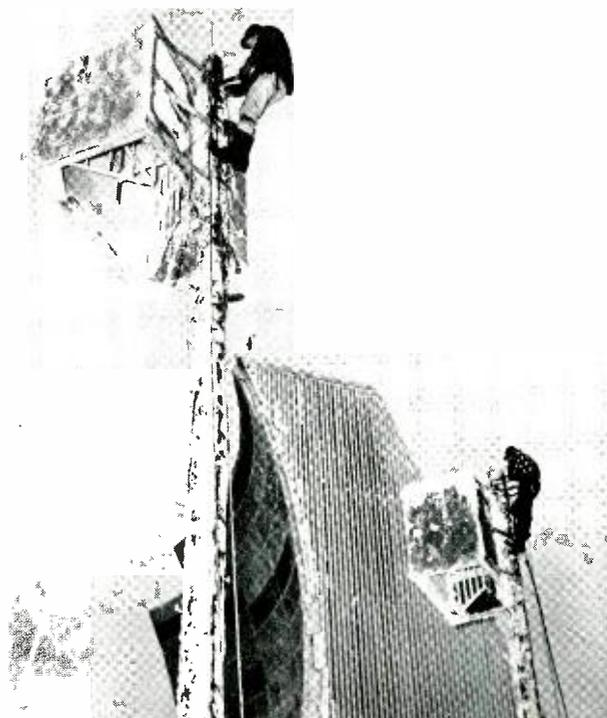
*Western Electric installation experts adjusting "side-leg" antennas at White Alice site. These small antennas provide communications to nearby points; large antenna is used for long distances.*
