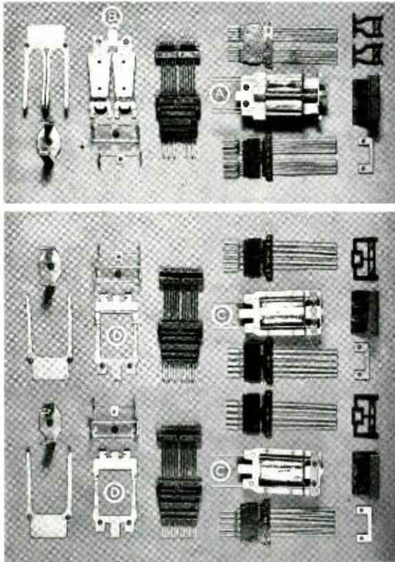
A striking comparison of the parts of the "two-in-one" relay (upper) with those of the two general-purpose relays formerly required to give an equivalent contact capacity for switching.
