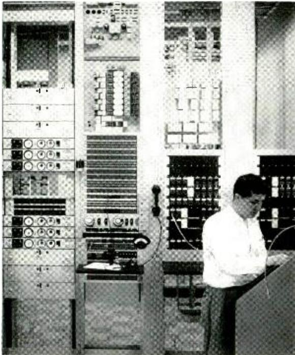
Part of the terminal equipment at Clarenville, Newfoundland. Bays at the left contain the monitoring equipment; the 92-kc pilots continuously monitor transmission between the cable terminals.
