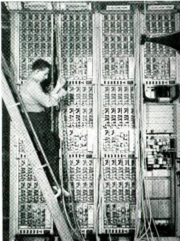
*An N1 carrier terminal installation. Extensive terminal equipment such as shown here makes carrier transmission costly for very short hauls.*
