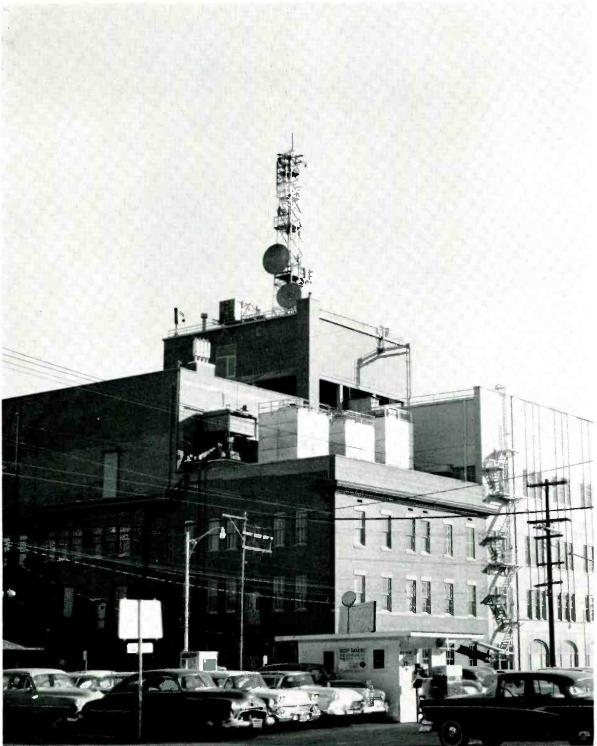
*This antenna tower atop a building in downtown Phoenix illustrates the variety of transmission media that serve a modern city. From the top: pole-type mobile-radio antenna, and dish-type antennas for radio-relay systems for television*
