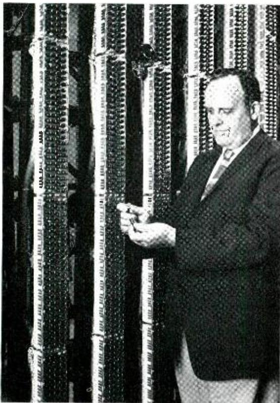
*At the Cockeysville, Maryland, trial installation, C. R. Noble demonstrates new cap and sleeve assembly. Each vertical row of connectors in this office protects up to 300 customer lines.*
