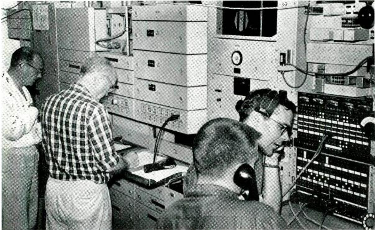
*Terminal equipment at repeater station along route of Canaveral Test Range communications system.*
