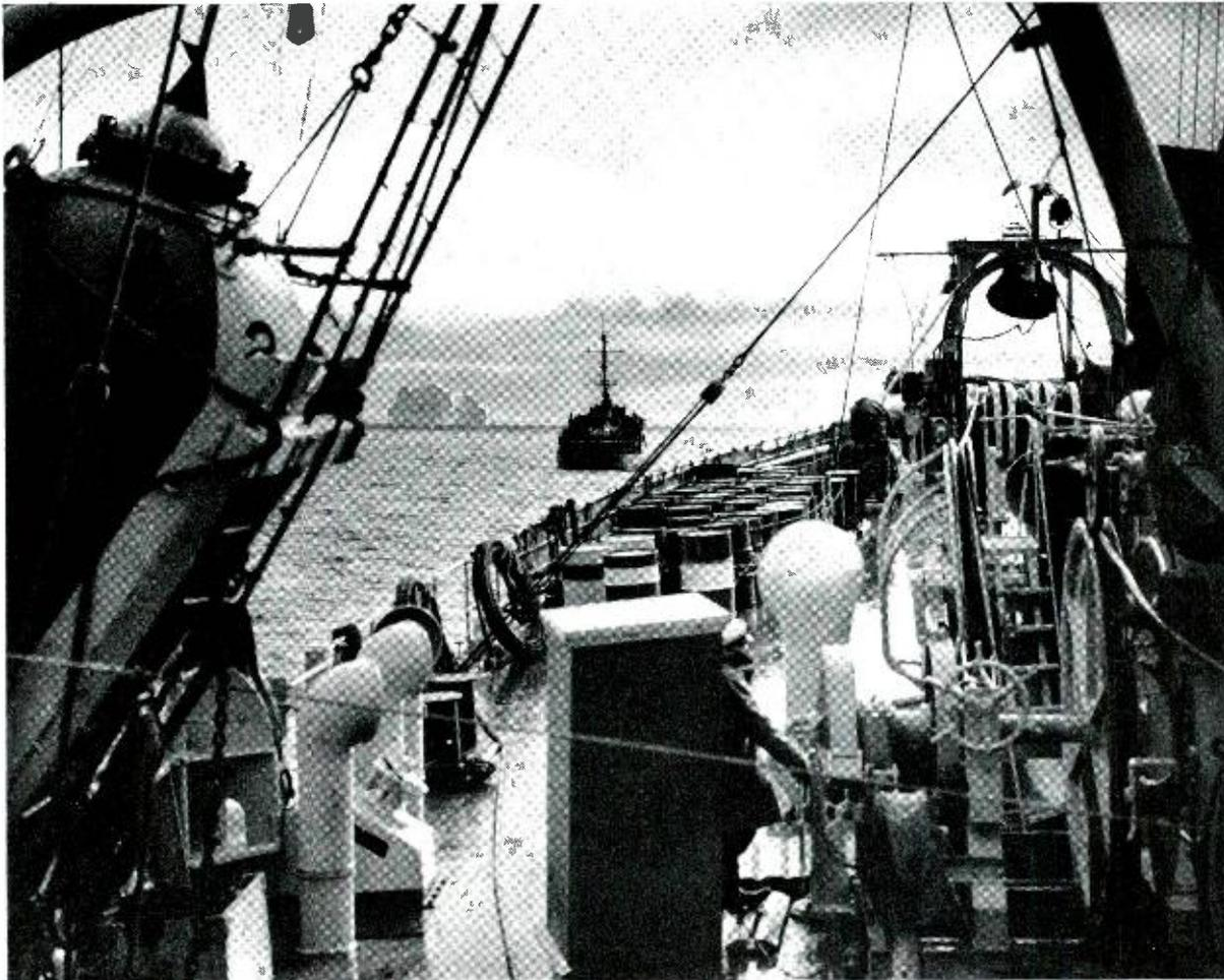
*Cable ship Monarch laying cable between Thule, Greenland and Canada. Installation of submarine*
