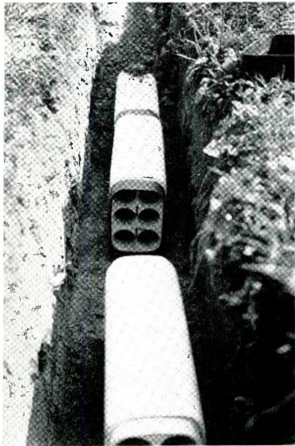
*Six-duct conduit sections with double tenon ends are aligned with dowel pins. A polyethylene sleeve provides a silt tight closure pad between each unit.*
