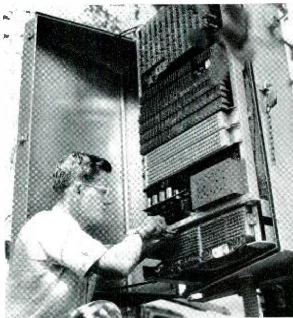
*R. Miller of New Jersey Bell Telephone Co. installing a 1A line concentrator at Martinsville, N. J.*
