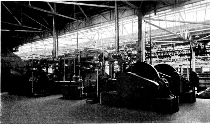
Fig. 16—Auxiliary equipment for vacuum driers.
