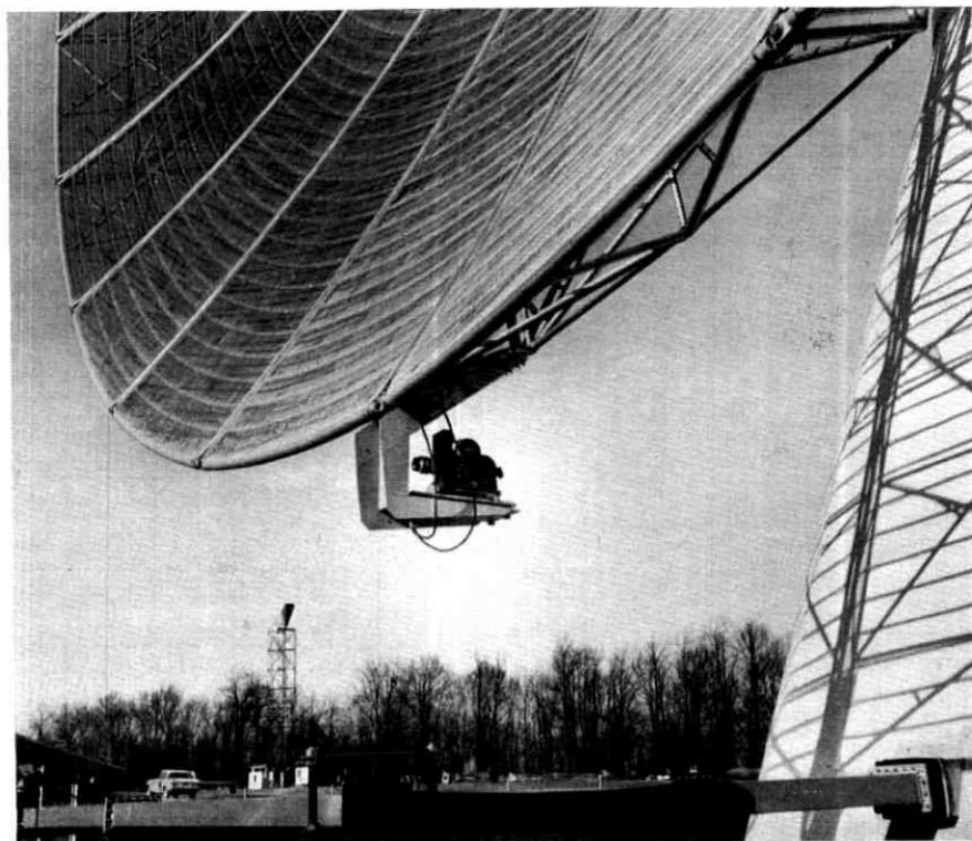
Fig. 5 — Camera mounted on paraboloid transmitter.
