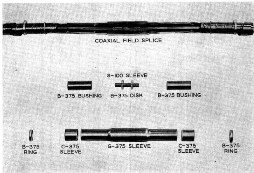
Fig. 9 — Coaxial field splice.
