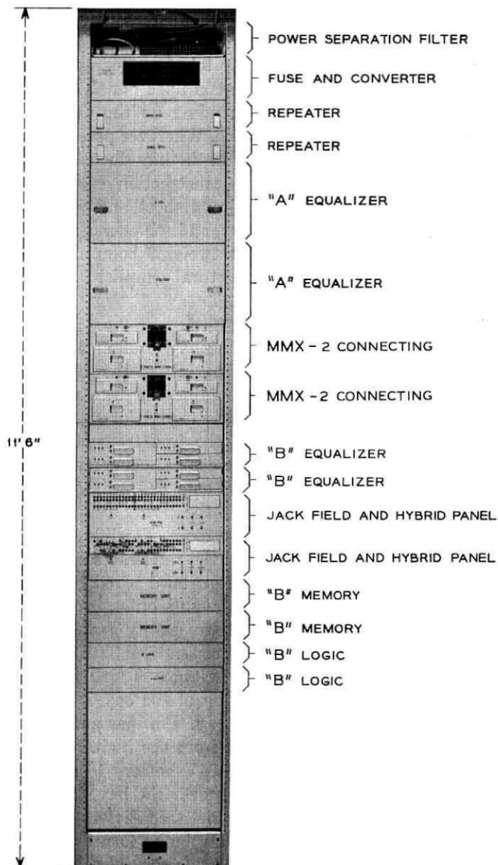
Fig. 39—Transmitting bay equipment arrangement.
