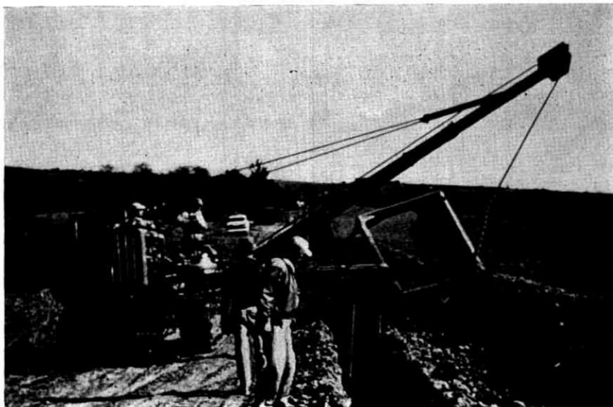
Fig. 8 — Backfilling and placing of shield wires.
