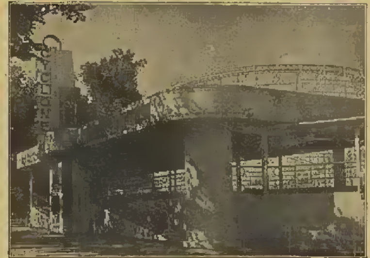
TOPPING THE RIDES in Lakeside Park, Denver, is the new Cyclone, 4,200-foot coaster built by Edward A. Vettel & Son, four miles of steel track, 50,000 bolts, 900 gallons of paint, 15 carloads of lumber and 150 kegs of nails were required to build the ride, which is said to incorporate every modern safety feature. Station is of glass brick, concrete and steel, has indirect neon lighting and specially designed ornamental iron rails with aluminum trim. Ticket office is of stainless steel, ornamental glass and interior lighted glass brick. An electrical signal system is set on a miniature painting of the coaster and lights indicate position of each train on the track. Trains pass thru a 250-foot enclosed tunnel.
