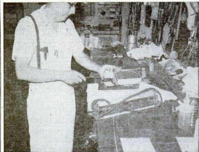
4. Selection system is virtually taken apart on the work table by E. Reinke in testing process. The four basic parts—selector, receiver pin assembly and front—are all given an individual treatment.
