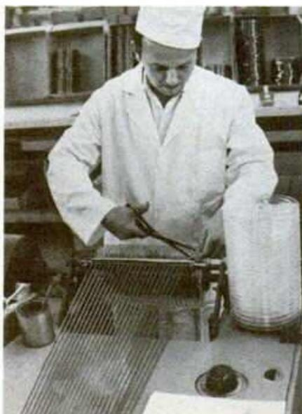
Separating lines of blank tape for open reel products.
