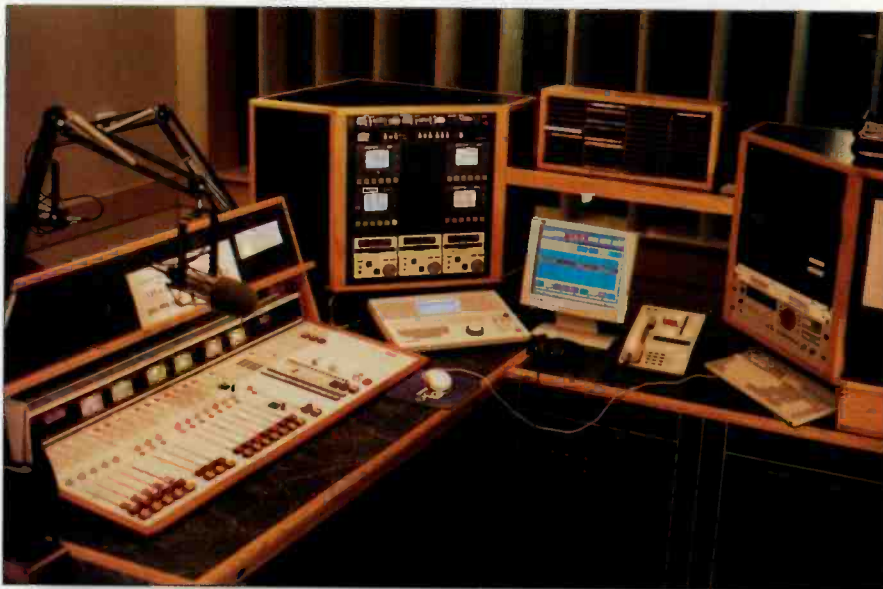
The space below racks provides a place to store equipment and supplies that are not in use. Photo by Connie Kramer.
