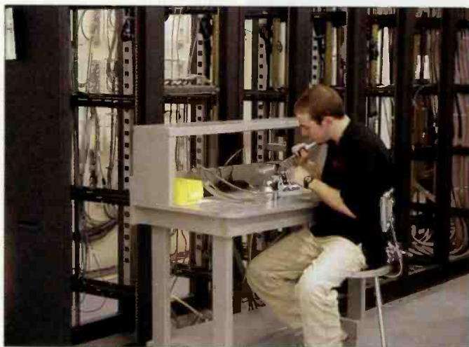
Constructing a facility requires extra labor.
