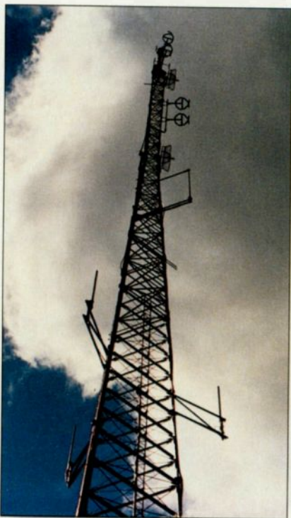
Tower inspections may require coordination with other tenants.
