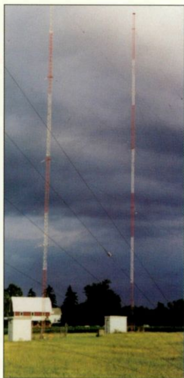
The tower itself is the RF radiator in AM applications.
