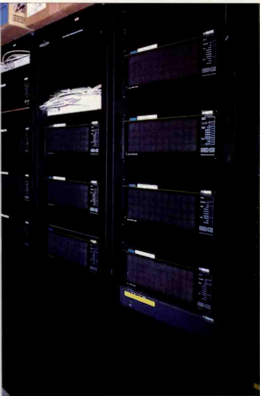
The Klotz Vadis audio routing frames at WCBS-AM, New York.
