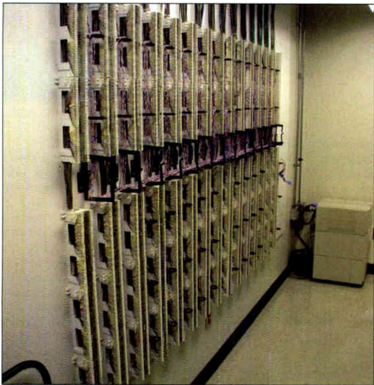
Originally installed for analog audio and signals, the wall of punch blocks sees little use now with so much digital audio and signaling.
