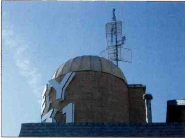
The grain silo isn't used to store grain anymore, but the natural height of the structure has another practical use for the station.
