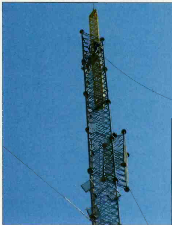
Stacking the tower sections.
