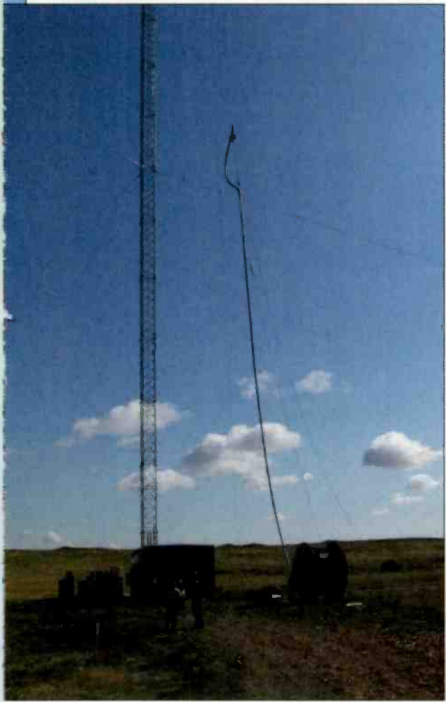
Hoisting the transmission line up the tower.
