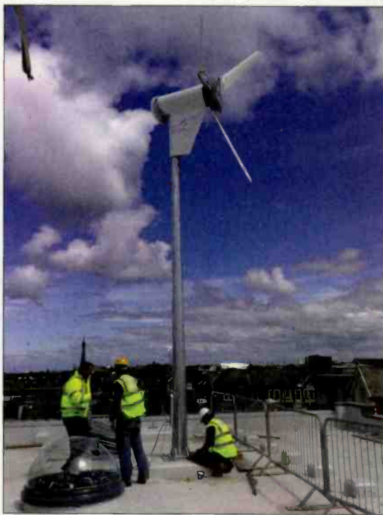
A Proven Engineering 2.5kW turbine mounted on a roof in Ashenden House, London.
