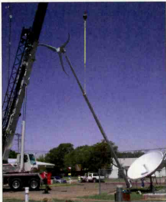
Hoisting the assembled KPAN turbine.
